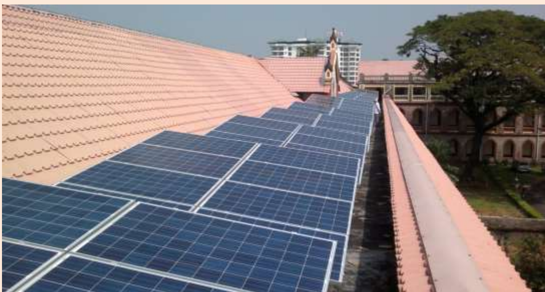
30kWp Grid connected Solar Power Plant at St Joseph Pontifical Seminary, Ernakulam
