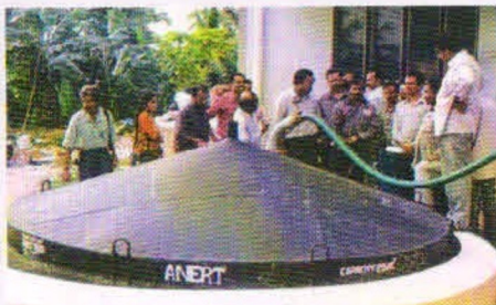
A 25m 3 Institutional Bio- gas Plant based on canteen waste installed at Hindustan Latex, Thiruvananthapuram
